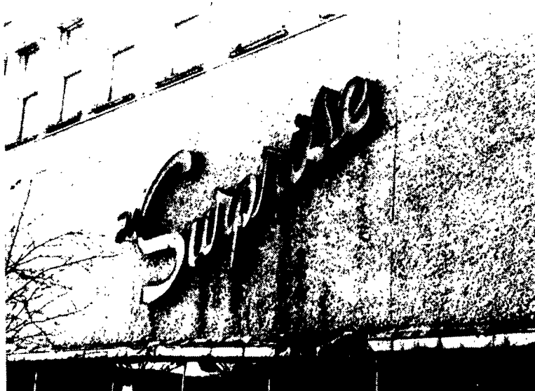
NEW LEASE ON LIFE? — Louis and Nancy Babbie hope to revive the old Surprise building, possibly with apartments and small boutiques.
