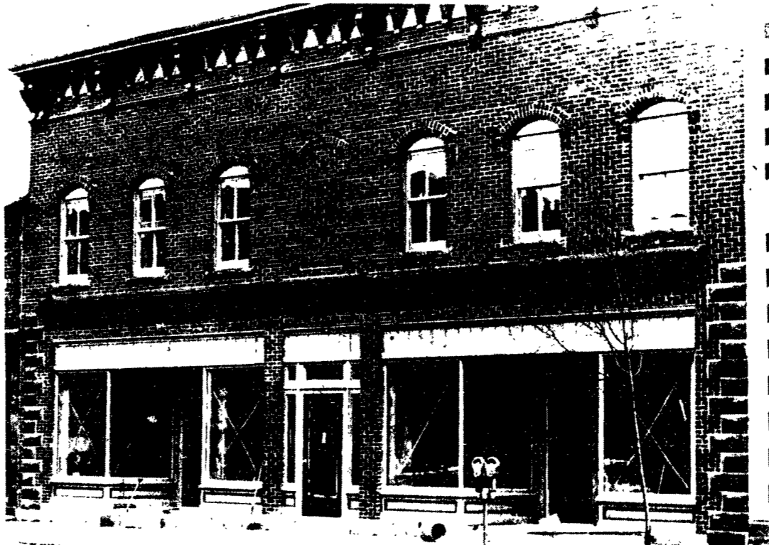
THE MARKETPLACE — Exterior facade work completed, work on the interior of The Marketplace, 26-28 Market St. is now continuing. The new building, a replacement for one destroyed by fire in January 1980, is part of a federally funded downtown improvement program. (Betsy Baker photo)
