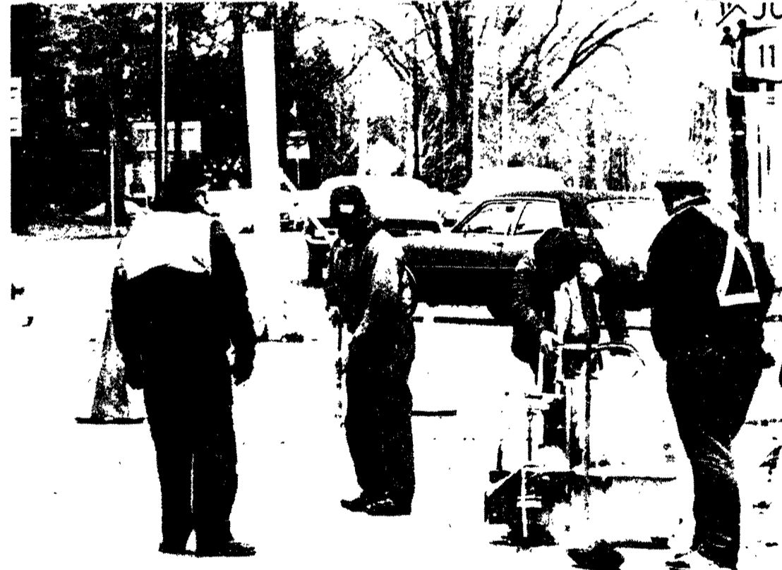
FINISHING TOUCHES — Construction workers finish up painting in preparation to the Nov. 19 opening of the Relief Route. (Bill Short photo)
