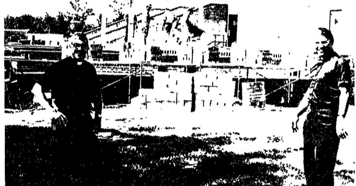
NEW LIBRARY ADDITION — The year 1979 brought a new library addition to Wadhams Hall Seminary. Here Rev. Richard Sturtz, Wadhams Hall librarian and Msgr. Peter R. Riani, college president, examine the construction of the new addition. The $300,000 project is being constructed by the Riverside Construction Company of Ogdensburg.
