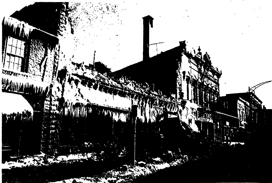
THE AFTERMATH—As one bystander put it, the east side of downtown Potsdam's Market Street Historic District looks like it had a tooth pulled. But for many, the pain that came with this extraction was more like heartache than toothache.
