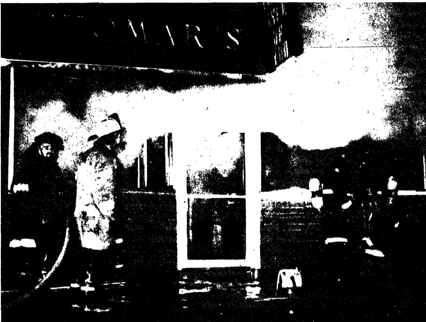
BUILDINGS DESTROYED —Look closely at the lower section of the glass door in the center of this photograph and you'll see the hole that has led to speculation that arson was behind a fire that burned through four businesses and two apartments at 26-28 Market Street in Potsdam early Thursday morning. Police launched an arson investigation after officers who first spotted the blaze at 2:55 a.m. stated that they saw this hole and another one in the glass door leading into the Thomaris Agency.
