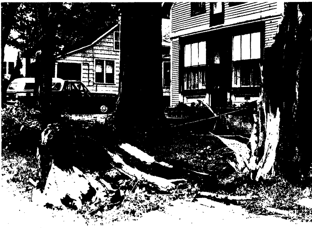
STORM DAMAGE —High winds followed by a driving rain storm on Saturday night caused trees, large limbs, and utility poles and wires to come down in West Stockholm. In the above photos, at upper left wires pulled a section of sliding away from the peak of the roof of this home owned by Elizabeth Brown of New Haven, Conn. At upper right, damage appeared most severe in front of the West Stockholm Post Office in background. At bottom, a section of this large tree brought down trees and utility poles in the yard of Mrs. Ruth Davis. (Hal Stokes photos).
