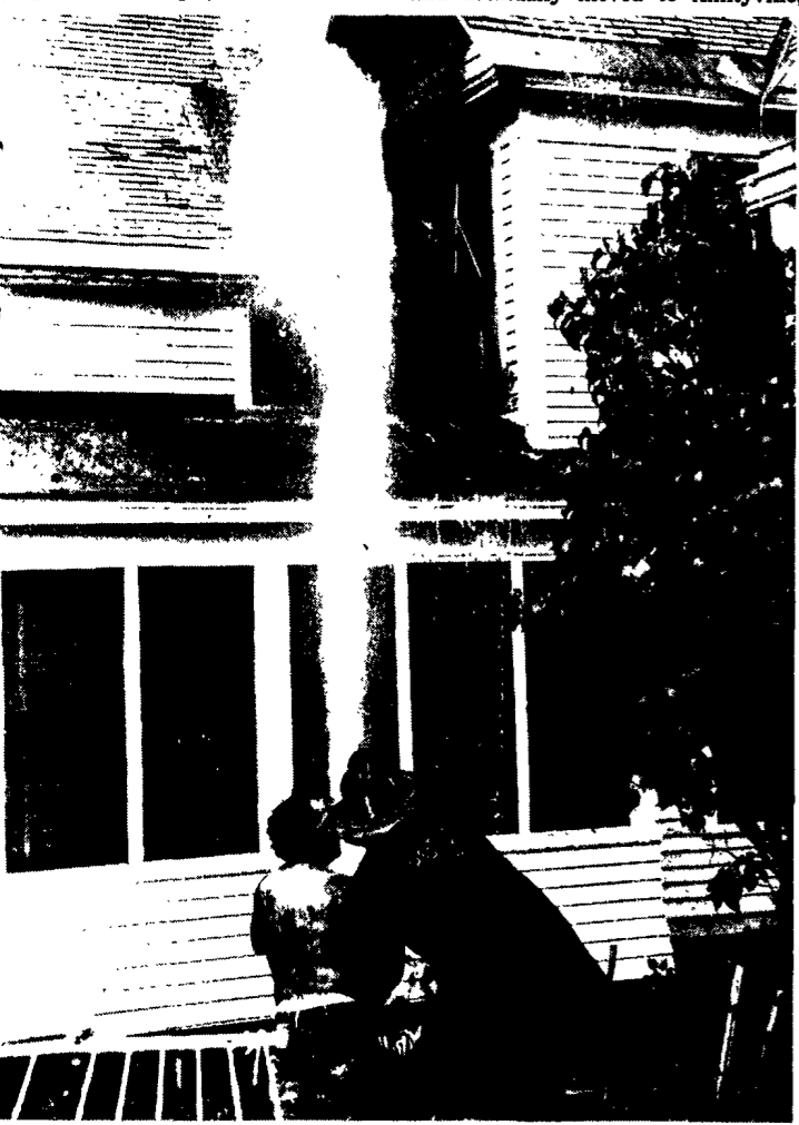
HOME DAMAGED—No official cause has been listed in a fire that caused heavy damage to the home of Allen S. Jones, 43 Pierrepont Ave. in Potsdam Monday afternoon. Potsdam volunteers responded to the blaze, which began in the attic of the two-story wood frame structure. Hannawa Falls firemen were on stand-by. A spokesman for the fire department said that there was an explosion, but that the fire was apparently well along prior to the explosion. (Betsy Baker photo).
