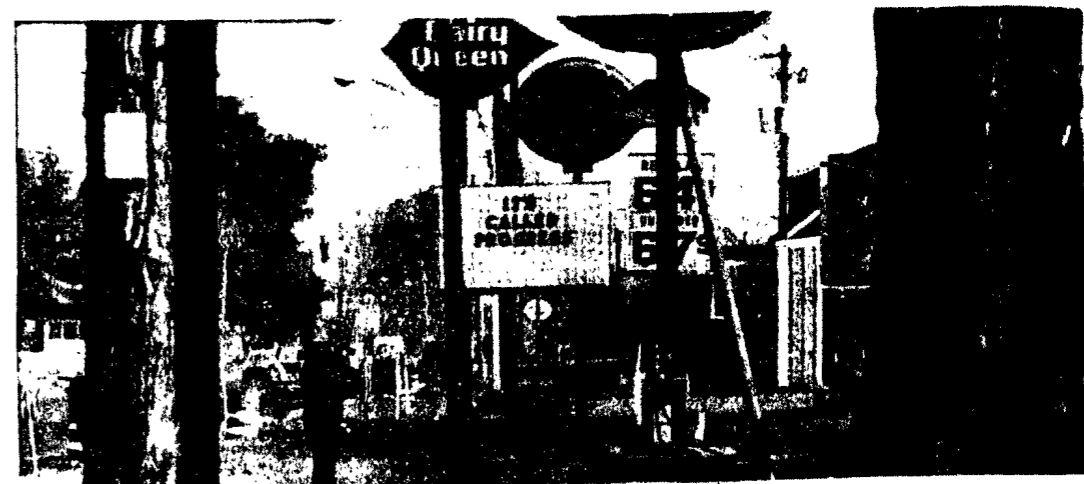
THE SIGNS SAY "It's called progress" outside the Potsdam Dairy Queen and it might not be ironic in nature. The outer section of Market Street in Potsdam has seen traffic tie-ups worthy of New York City this summer as a result of a road widening project. (Mike Billington Photo)
