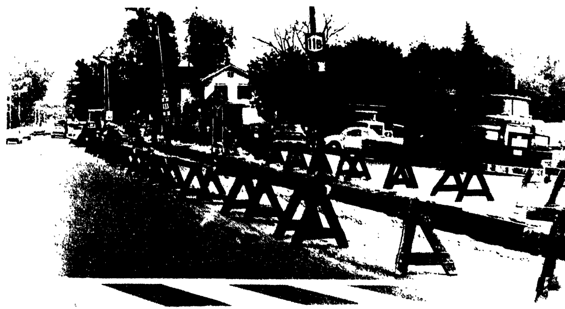
NO, IT ISN'T the Alaska Pipeline...but it is site improvement work along Main Street in the Village of Potsdam. JVL Construction Company landed the Urban Renewal Agency contract which also includes work in Ives Park and both sides of Market Street. (Will Brady Photo).
