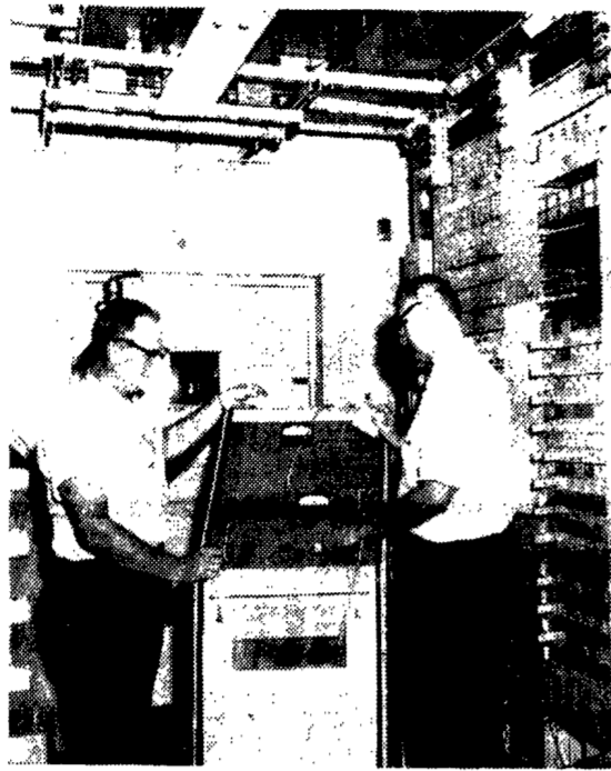
FINAL CHECK — New York Telephone plant manager Fred Stone (left) and switchman Paul Boatman test equipment at the company's central office in Potsdam, which will have a "cutover" to direct distance dialing for telephone customers in this area early Sunday morning.
