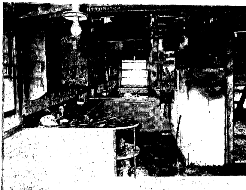
KITCHEN IN RUINS — Here's how the kitchen in the Robert Barstow home on the May Road looked after fire swept through the house last Sunday morning. An explosion from the garage caused flames to sweep across the kitchen ceiling. The kitchen and garage were completely destroyed and smoke and water damage were extensive in the rest of the house. —Photo by Laird Chaffee
