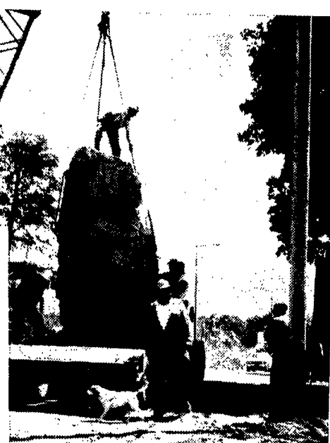
seems to be what the workman is saying as he stands just after the 35-ton granite boulder has just been lifted from its resting place and swung over to the flat bed truck in the foreground for movement over a half hour for the workers to adjust the cables they released the heavy cable chains.
