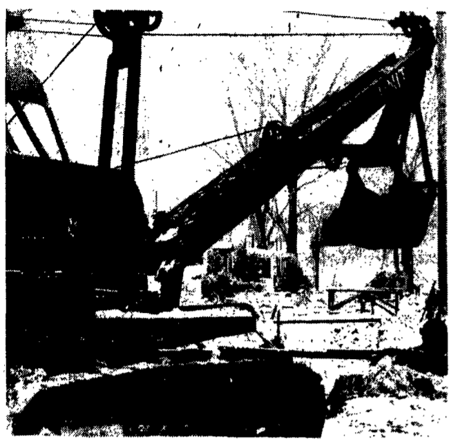
This power shovel, at work on the Barclay St. storm sewer project, was joined by another shovel this week in response to protests from village officials. Work was progressing slowly and Carson James, village street superintendent notified a state inspector that it was creating a hazard because fire trucks could not use the street. Another shovel was put on the job on Monday on the sewer, which will connect with the new Potsdam State Teachers College campus.
