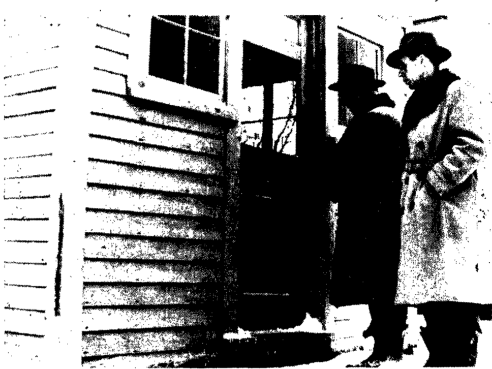
James T. Lahey, Potsdam civil defense director, opens the door to the air raid lookout post atop the village filter plant as Grant Cotton, chief observer, stands by. The men inspected the post this week to see what installation would be needed to reactivate it.
