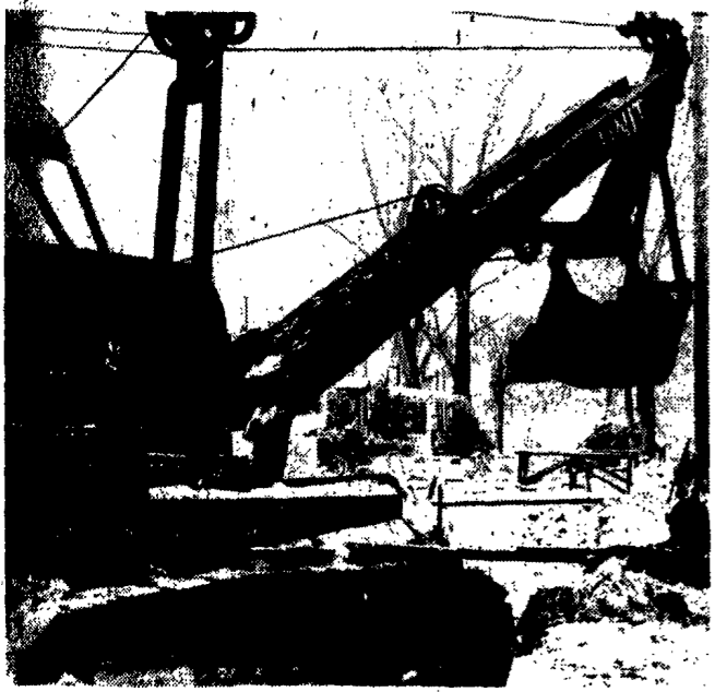
—Courier and Freeman Photo by Dennis Webster This power shovel, at work on the Barclay St. storm sewer project, was joined by another shovel this week in response to protests from village officials. Work was progressing slowly and Carson James, village street superintendent notified a state inspector that it was creating a hazard because fire trucks could not use the street. Another shovel was put on the job on Monday on the sewer, which will connect with the new Potsdam State Teachers College campus.
